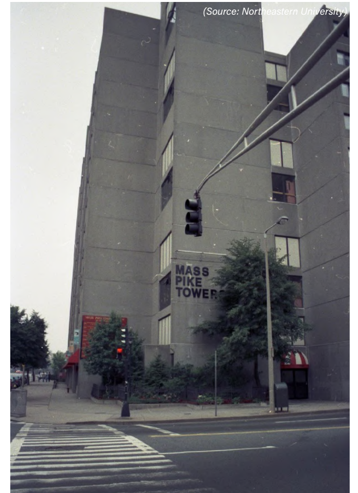
1970s: The towers stand proud shortly after completion.
