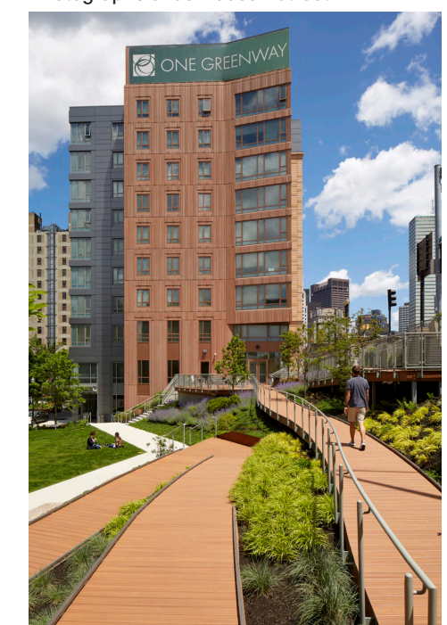
Photographs of 66 Hudson Street
